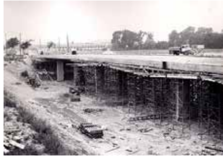
On 8 February 1972, the day before the official opening, the Fiskebæk bridge collapsed. Without warning, the western motorway flyover fell into the bog. Even though no one was hurt in the accident, the collapse may have made its mark on Danish foundation standards. Photos: Vejdirektoratet.
