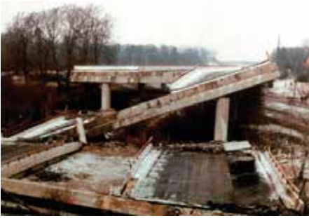
On 8 February 1972, the day before the official opening, the Fiskebæk bridge collapsed. Without warning, the western motorway flyover fell into the bog. Even though no one was hurt in the accident, the collapse may have made its mark on Danish foundation standards. Photos: Vejdirektoratet.
