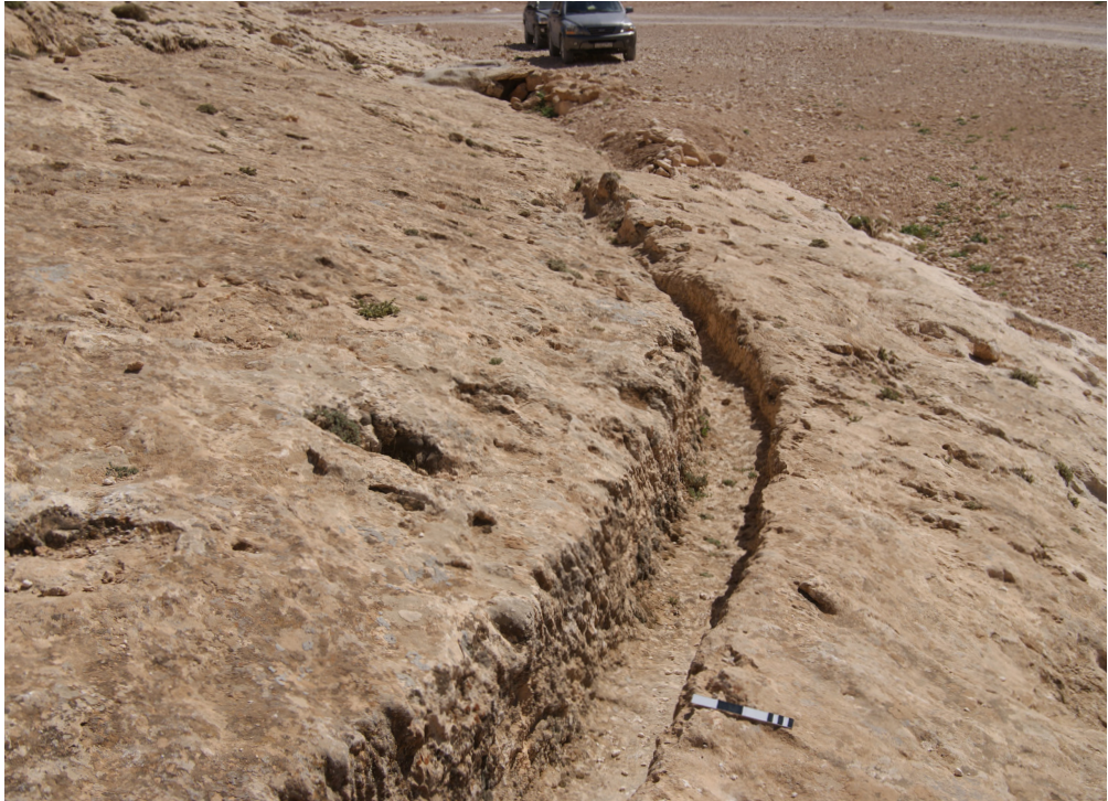
Fig. 4: Cistern site with a carved channel, curving across the rock to catch rainwater runoff (Copyright: Jørgen Christian Meyer).
