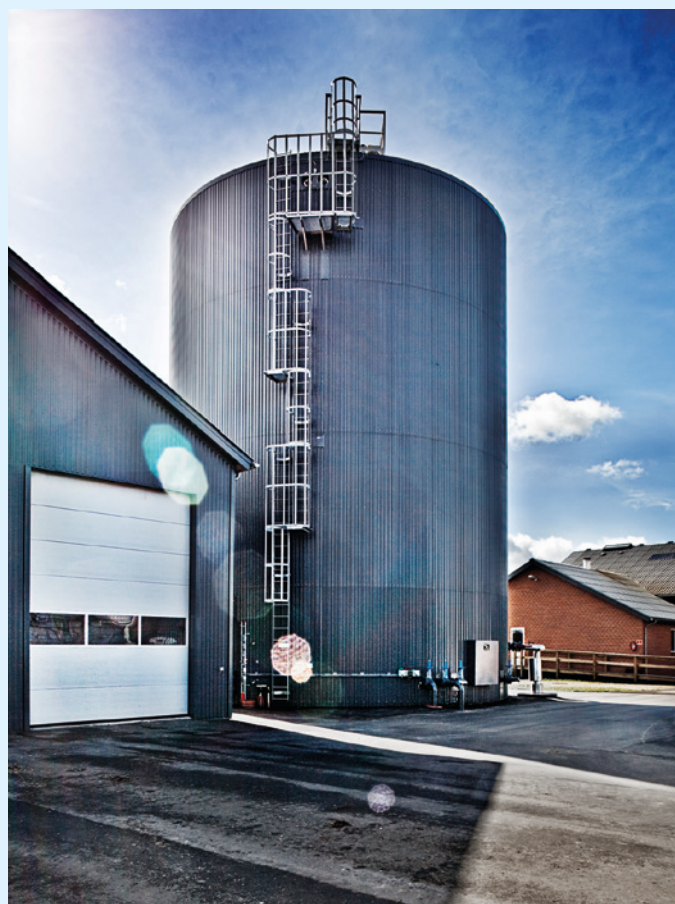
The Biogas plant at Aarhus University
